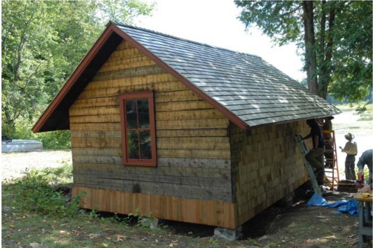
Lake Harris Boat House under restoration (2012)
